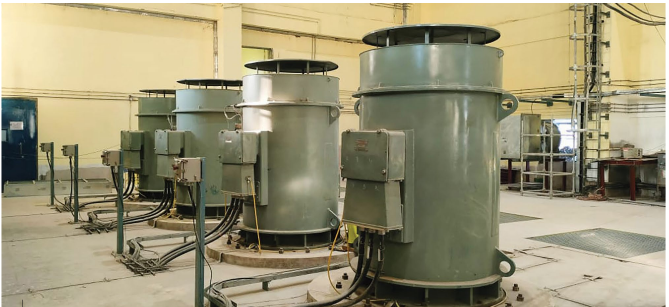
Metallic Volute Pumps (MVP) supplied to a nuclear power plant in Rajasthan
